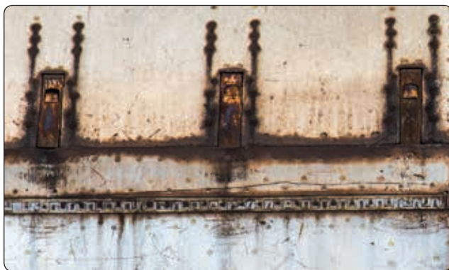
Figure 8-18. Galvanic corrosion.
